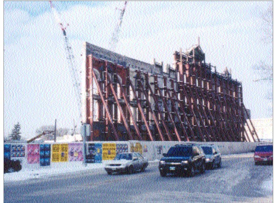
Above: Work underway, as of January, 2002
