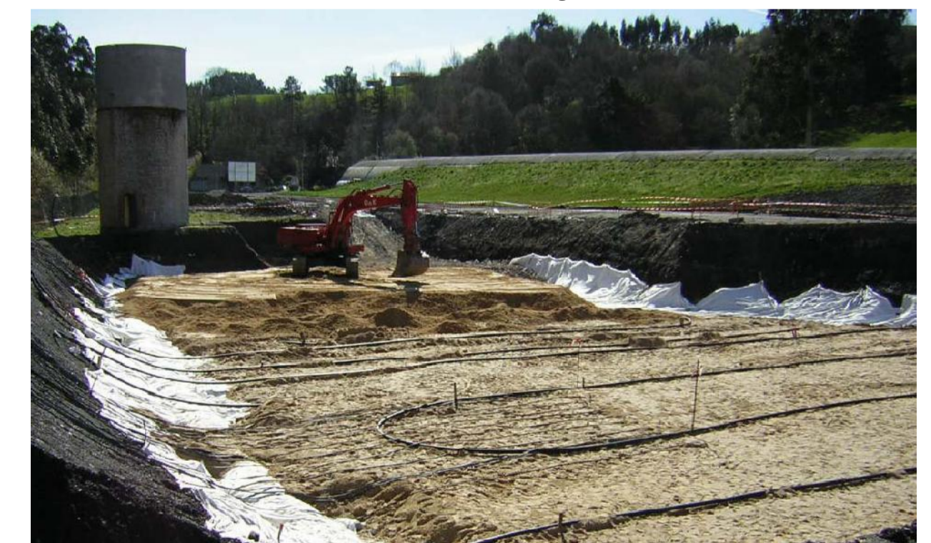
Geothermal heat recovery
