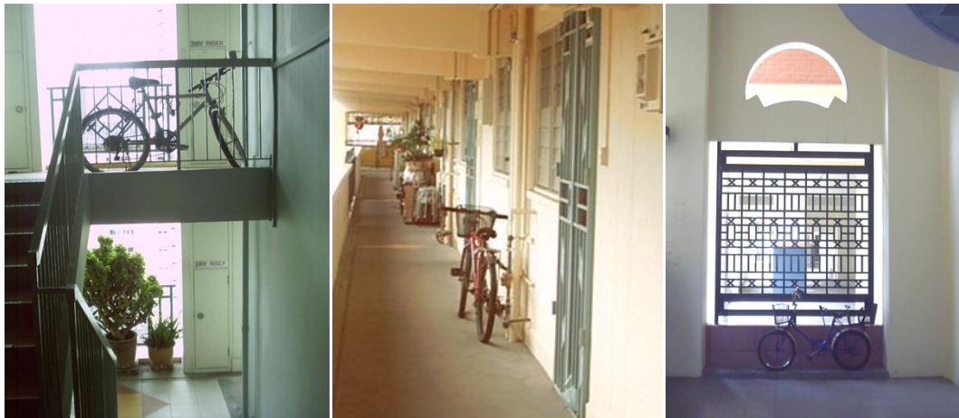
Figure 7: The presence of bicycles at staircase handrail, common corridor, and void-deck.
