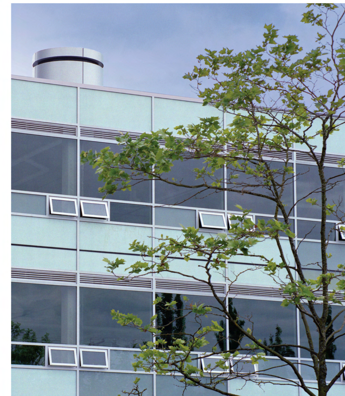
The north façade features horizontal louvers, operable windows and high performance glazing
