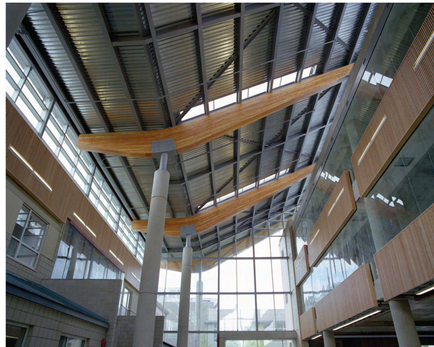
Large curved glulam beams are the focal point of the three storey atrium space for the new Administration Building. The light-filled atrium bridges the gap between the old and the new buildings
