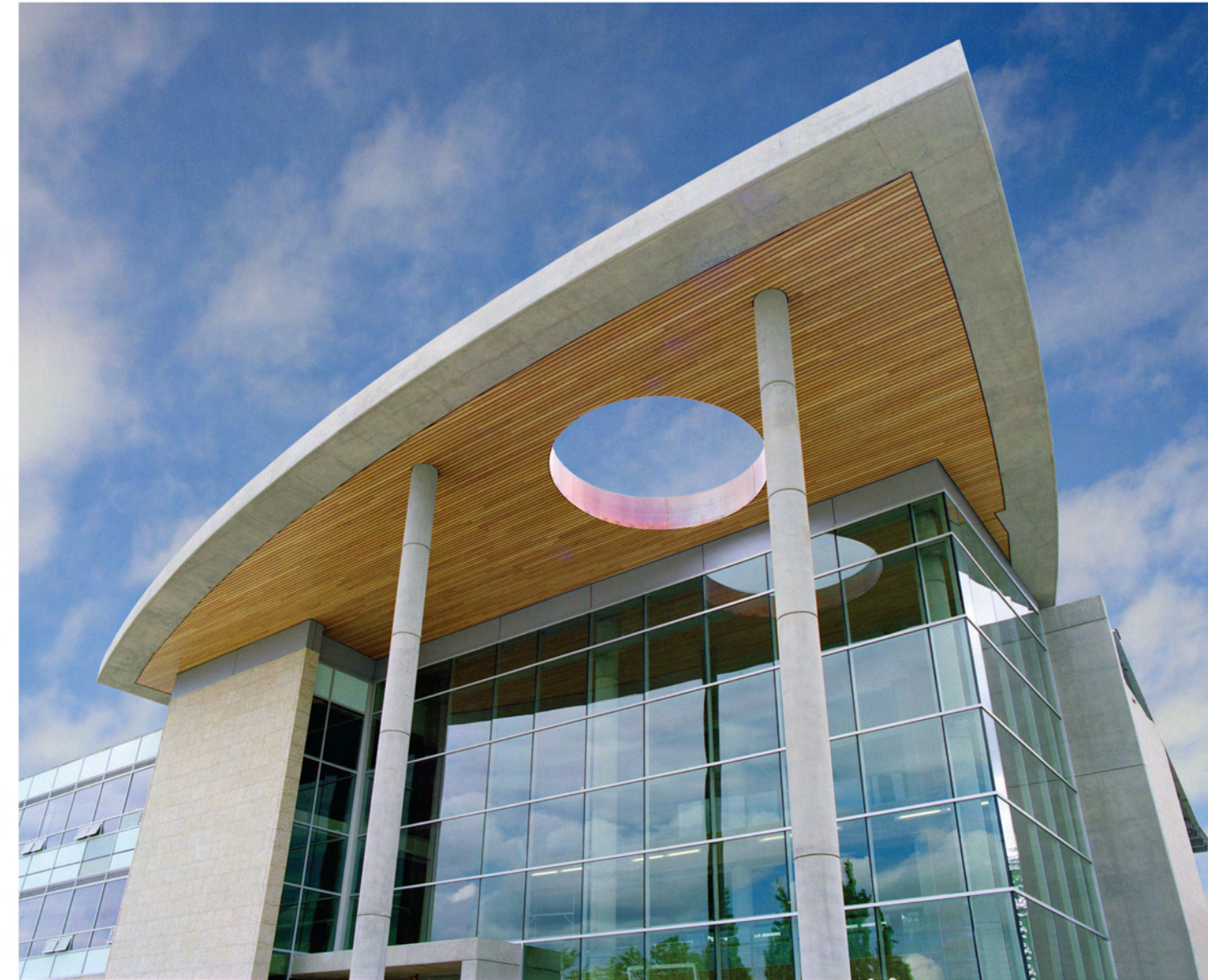
The new entrance features a dramatic canopy with copper ringed oculus and wood soffit
