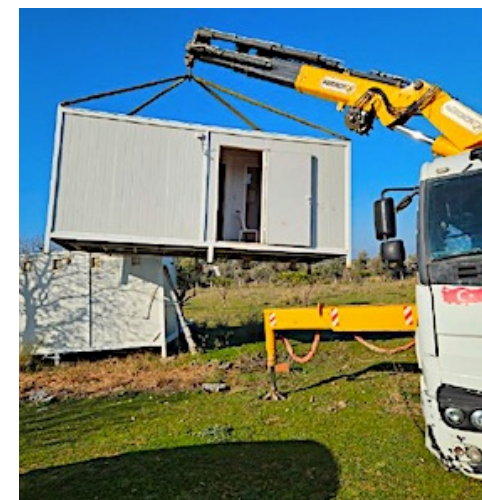
Toilet and shower modules sent to Iskenderun
