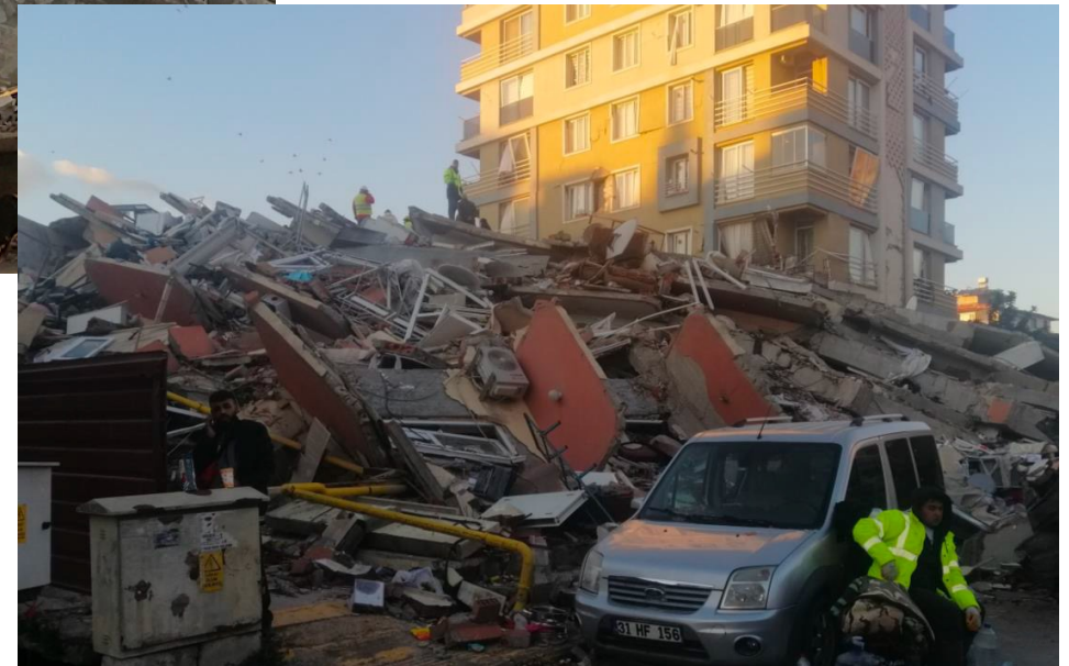
Earthquake zone, Feb. 6-7 (Dr. Ilker Kahraman) Note that some buildings remain intact while others collapse completely
